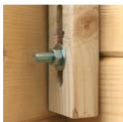
Storm braces (log pavilions)
